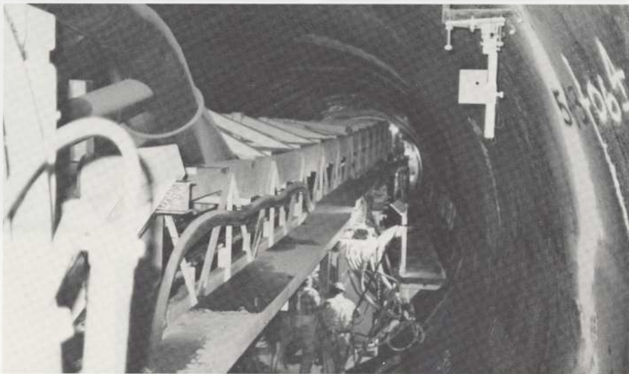
Robbins tunnel boring machine carving out an 8-mile long, 18-foot diameter tunnel.
