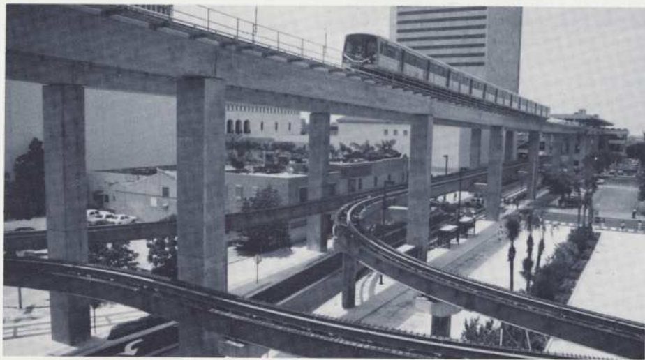
The prestressed concrete box girders carrying the Miami Metrorail train and, below, the partially completed guideway structures for the Downtown People Mover.
