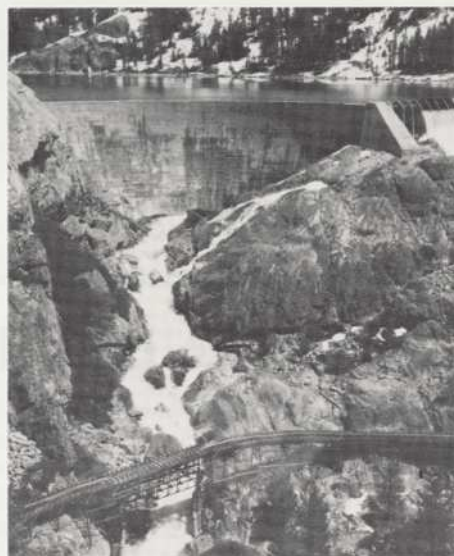
Bowman Lake's South Dam and Spillway caught during a Spring spill. The remnants of the old Bowman-Spaulding flume — now abandoned and replaced by a tunnel — are seen in the foreground.
