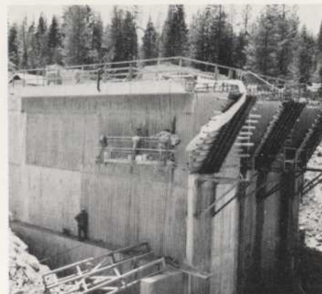
Jones Fork Power Plant, concrete top out
