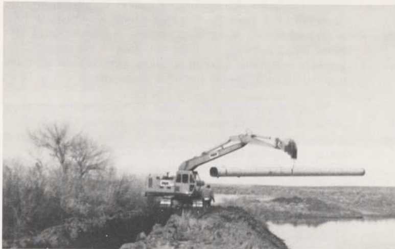
Laying pipeline at Duck Valley
