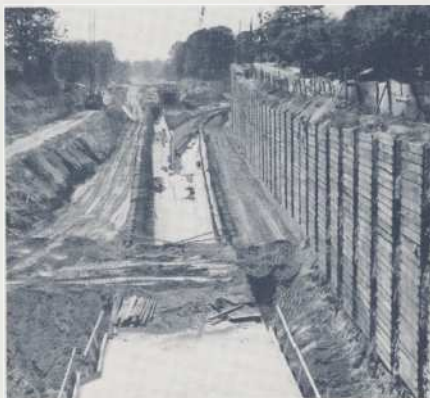
Subway construction in open trench on the MARTA West Line - "Y" visible in background
