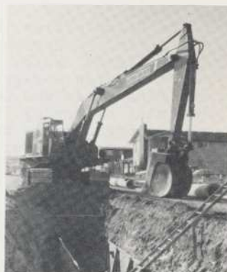
3CY bucket backhoe over 16 foot deep trench.
