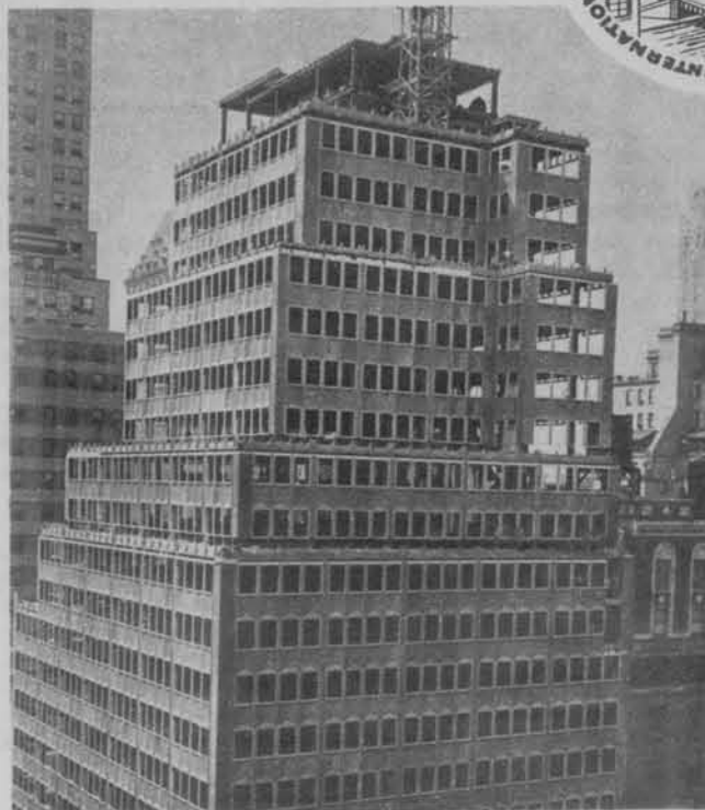
Curtain wall construction.
