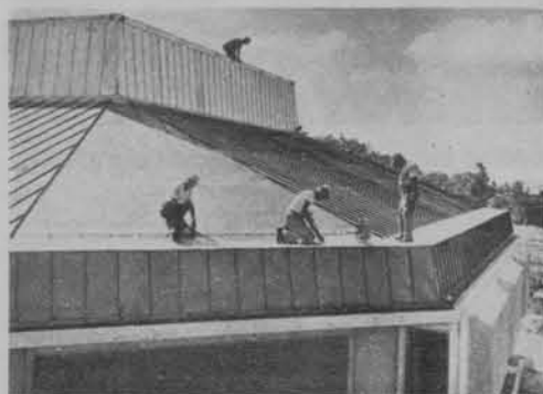
Sheet metal roofing is a traditional skill and it keeps pace with building changes. I.A. men work in both metals and plastics.
