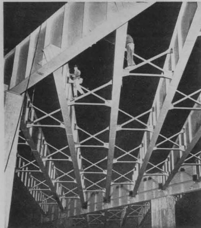
Night work on a highway bridge to avoid day time traffic.
