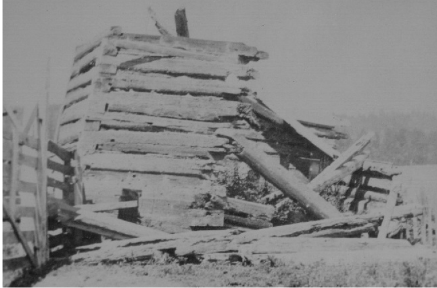
Figure 4. Blockade bastion with earthquake damage, ca. 1910. Catalog # 090-4534.
