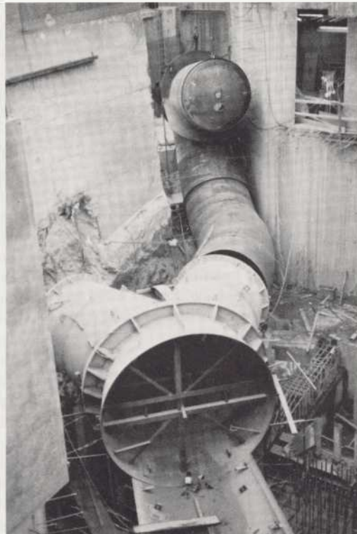
Upper left and above — Friant-Kern No. 1 turbine case Y-branch installation Lower left — River outlet horizontal Francis turbine
