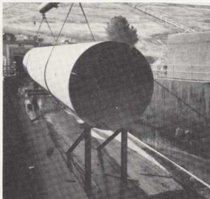
160-foot section of steel tunnel liner.
