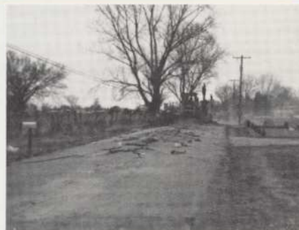
Lifted road surface after blasting.
