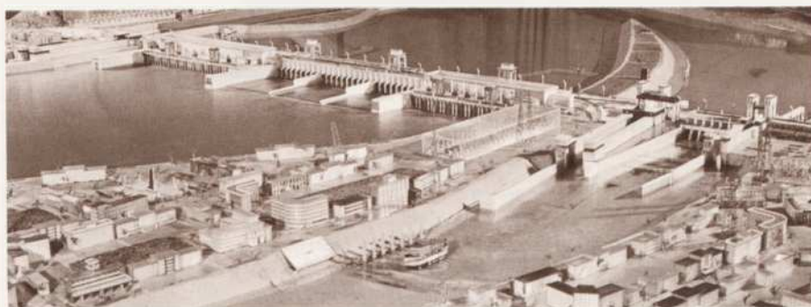
Working model of the Gezhouba Dam. The ships move up into the ship locks in this model.
