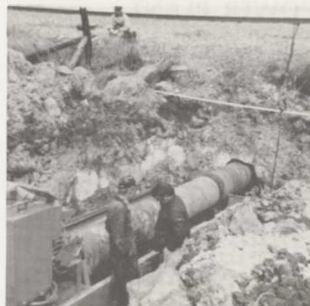
Installation of 24" steel casing under railroad tracks through solid rock. A circular bit is welded to the end of the casing and the rock is removed in the form of a core.
