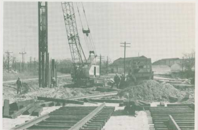
Rail relocation and pile driving for the Arizona Avenue Underpass
