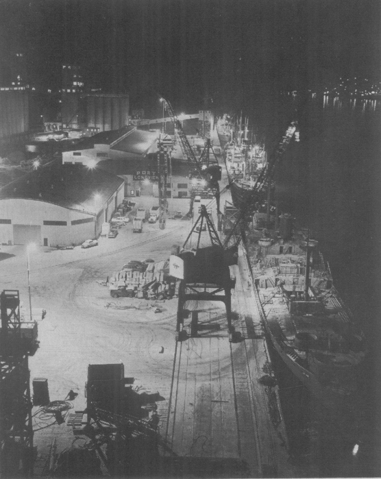
Mechanized dock at Longview, Washington. The office and warehouse in the center have been removed to permit the 65 and 70-ton whirley cranes to serve three ships' berths.
